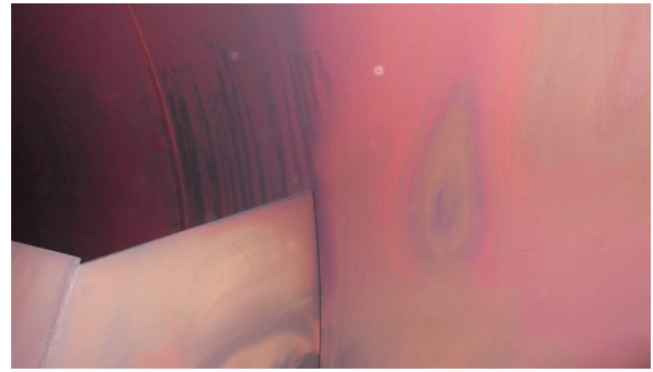
Figure 2: LP drum after OEM chemistry optimization
